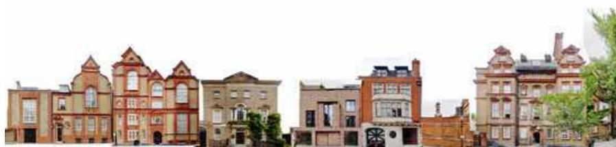
Photo montages of No. 31 to No. 3 Tite Street
